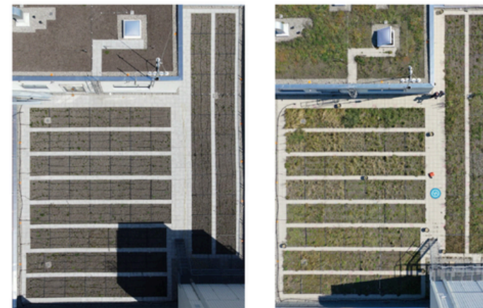
The roof in August 2020 and 2022
